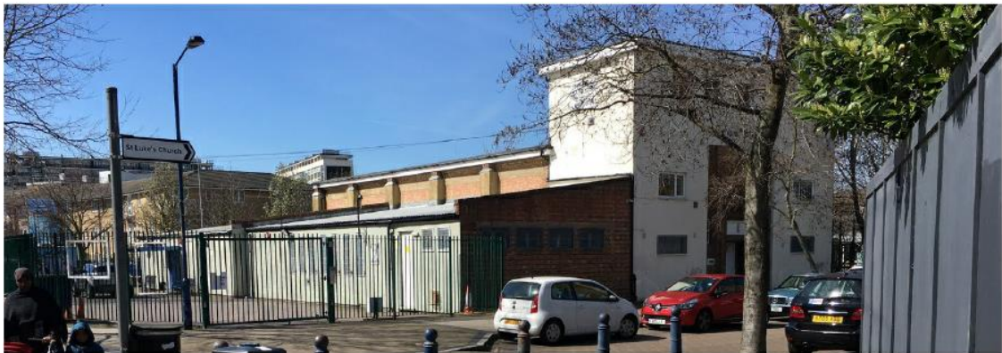
Existing Bradfield Youth Club seen from Commercial Way, looking west
